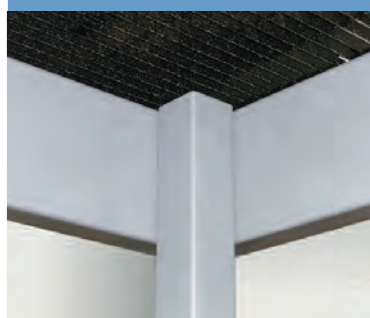
▲ The Strongbox beam-to-column connection completely eliminates the need for gussets.
